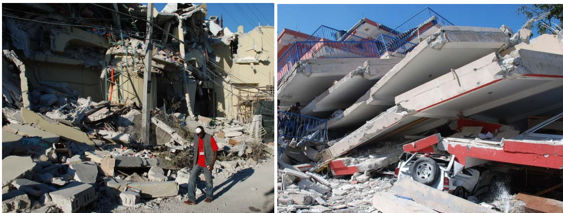
Figure 5. Urban destruction following 2010 Haiti Earthquake (IFRC, 2012)
